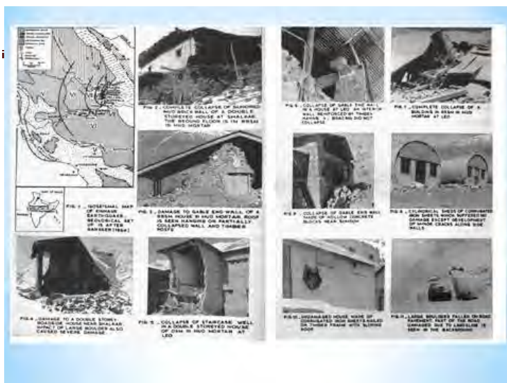
Figure 14: Physical Damage Pictures of 1975 Kinnaur Earthquake
