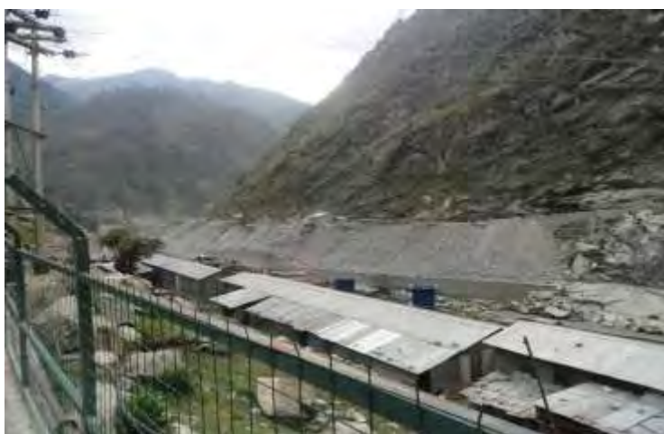
Figure 8: Unscientific Dumping of Muck along the natural course of river
