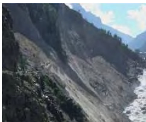
Figure 21: Loss of road and landslides
