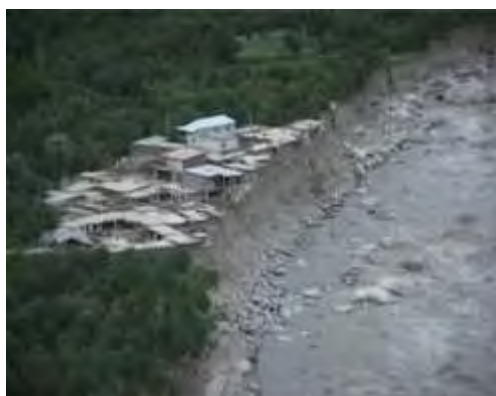
Figure 20: 2005 Flood: Damage to Leo Village
