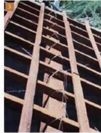
Connection of purlins & rafters, and beam & rafters.
