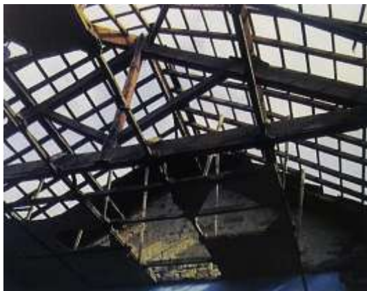
Damage to light roof due to cyclone
