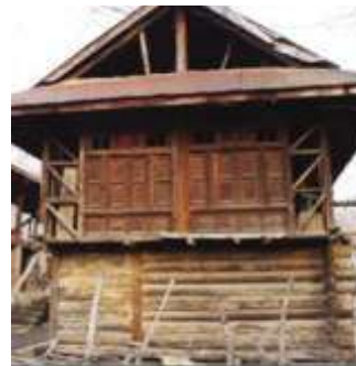
Timber walls with CGI sheets hipped roof- Jammu & Kashmir
