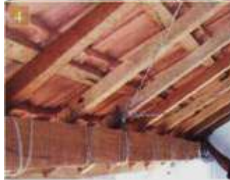
Connection of purlins & rafters, and beam & rafters.
