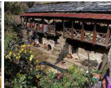
Ashlar Stone Walls with shingle gable roof - Jammu & Kashmir
