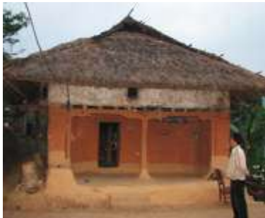
Adobe walls with thatch hipped roof - Sikkim
