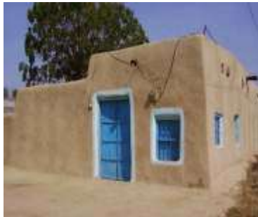
Adobe walls with timber & mud flat roof - Haryana
