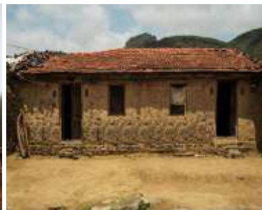
Stone rubble masonry walls with country tile flat roof- Dadra and Nagar Haveli
