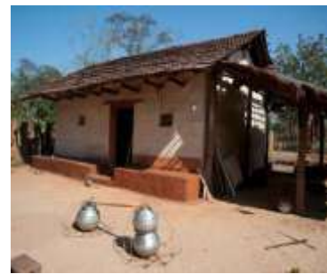
Wattle and daub walls with Mangalore tiles gabled roof - Odisha
