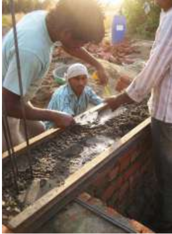
C8 Hazard Resistant Features for Foundation and Plinth NDMA Unnati PIC
