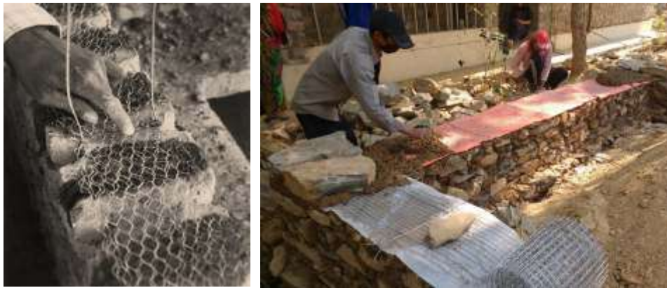
Weld mesh encased in 25 mm thick layer of mud mortar.
