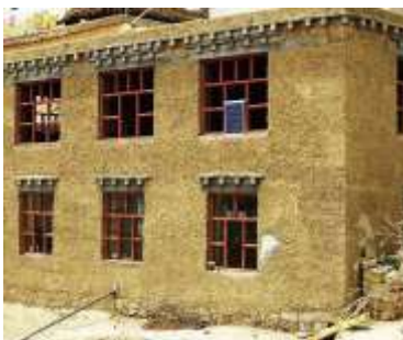
Adobe walls with timber & mud flat roof - Himachal Pradesh
