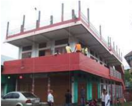
Burnt Brick walls with RCC flat roof- Haryana
