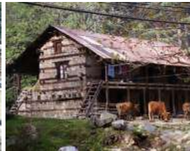
Stone rubble masonry walls with CGI sheets gabled roof- Himachal Pradesh
