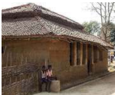
Cob walls with tiled hipped roof - Chhattisgarh
