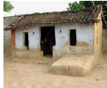
Adobe walls with country tiles gabled roof - Rajasthan
