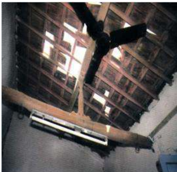
C3 Hazards: Their Severity, Zonation and Impact on buildings NDMA Unnati PIC
