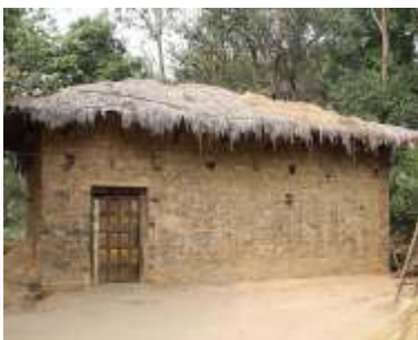
Stone rubble masonry walls with thatch hipped roof- Jharkhand
