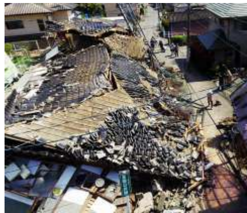
Damage to heavy roof due to earthquake
