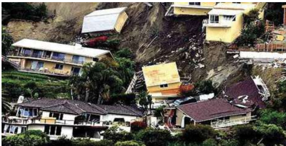
C3 Hazards: Their Severity, Zonation and Impact on buildings NDMA Unnati PIC
