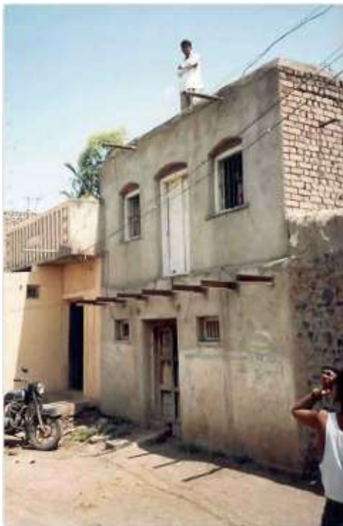
Burnt Brick walls with RCC flat roof- Uttar Pradesh
