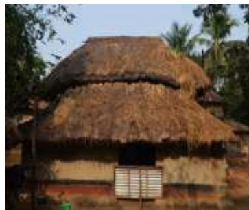
Cob walls with thatch hipped roof - West Bengal
