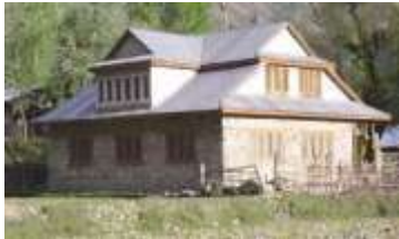
Stone rubble masonry walls with CGI sheets gabled roof- Jammu & Kashmir
