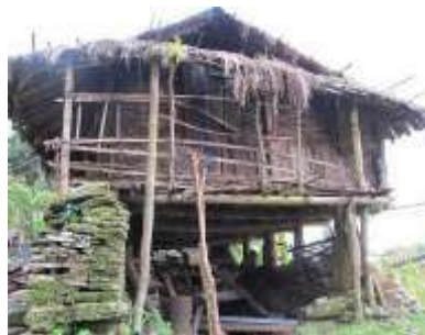
Timber walls with thatch hipped roof- Sikkim
