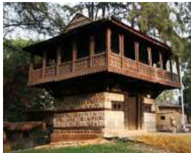
Ashlar Stone Walls with CGI sheets hipped roof- Himachal Pradesh
