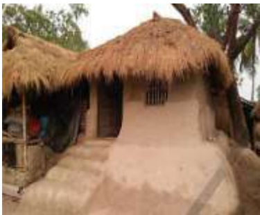
Adobe walls with thatch hipped roof - West Bengal
