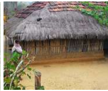
Wattle and daub walls with thatch/ filed hipped roof - Jharkhand
