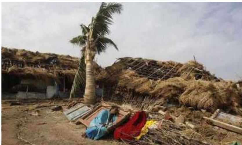
Severe damage to load bearing structures
