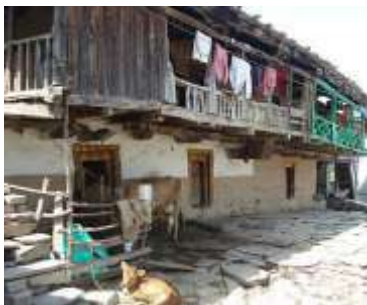
Timber walls with timber gabled roof- Uttarakhand
