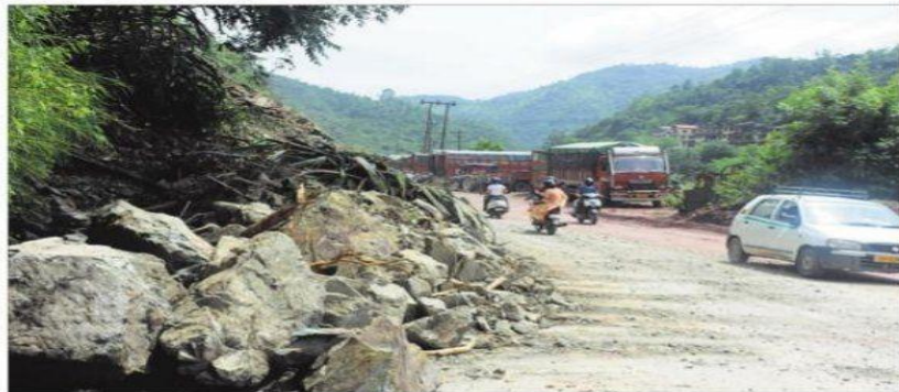
A landslide on the Chandigarh-Manali national highway near Mandi. PHOTO: JAI KUMAR
