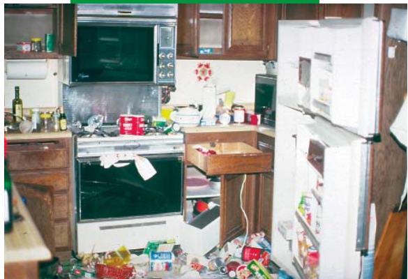
Top: Structure shifted on its foundation in Watsonville, Calif. Bottom: Nonstructural kitchen damage, Northridge, Calif.
