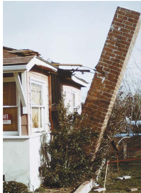
Chimney damage, San Fernando, Calif.
