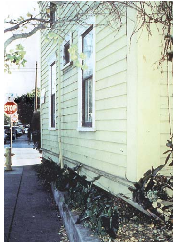
Cripple wall foundation failure, Northridge, Calif.
