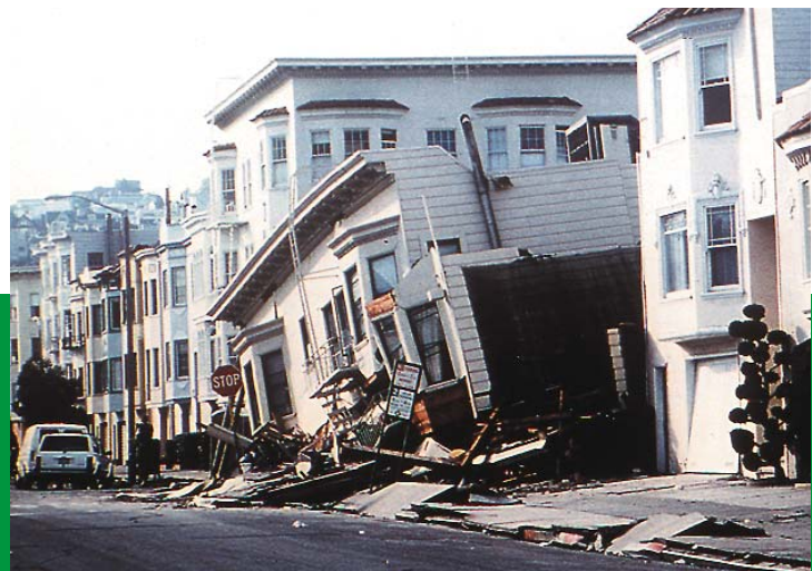
Damage in San Francisco's Marina District.
