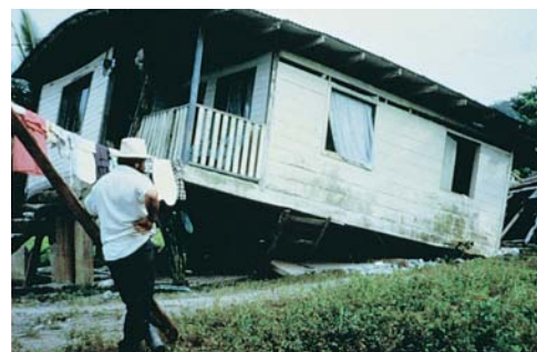
Post-and-Pier Foundation; undamaged (top) and damaged (bottom), Costa Rica.
