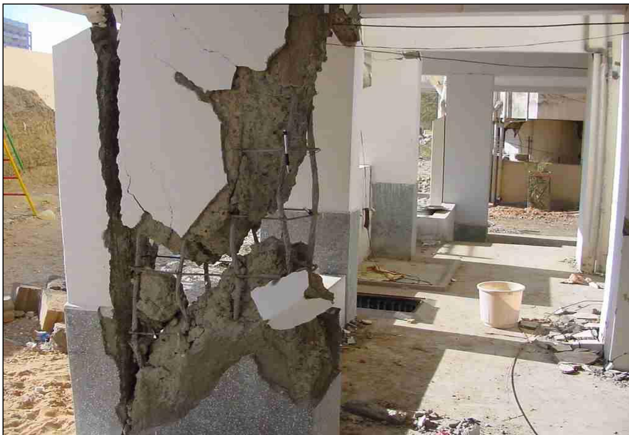
Figure 6: 230 mm wide columns in ground storey of RC Frame Buildings: damaged column in Bhuj town during 2001 Bhuj earthquake
