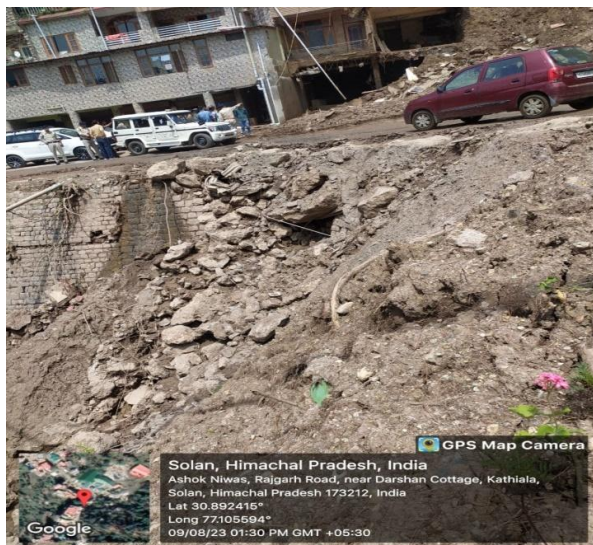
Figure 4 Location before disaster
