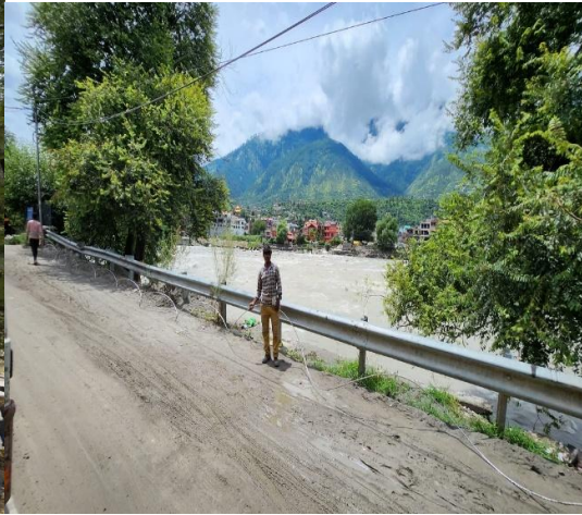
Figure 13 Restoration Work In Progress
