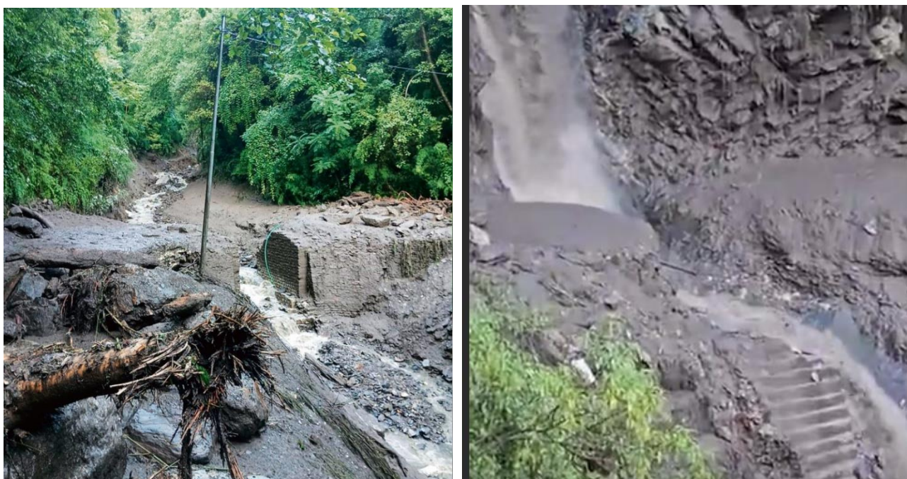
Damage caused by cloud burst at Taklech Nala
