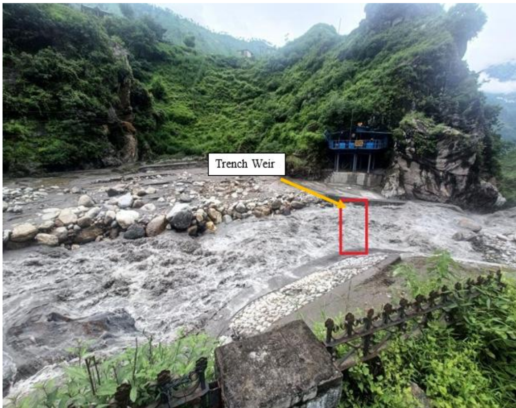
Figure 2 Flow over trench weir of Ganvi Project Stage-I
