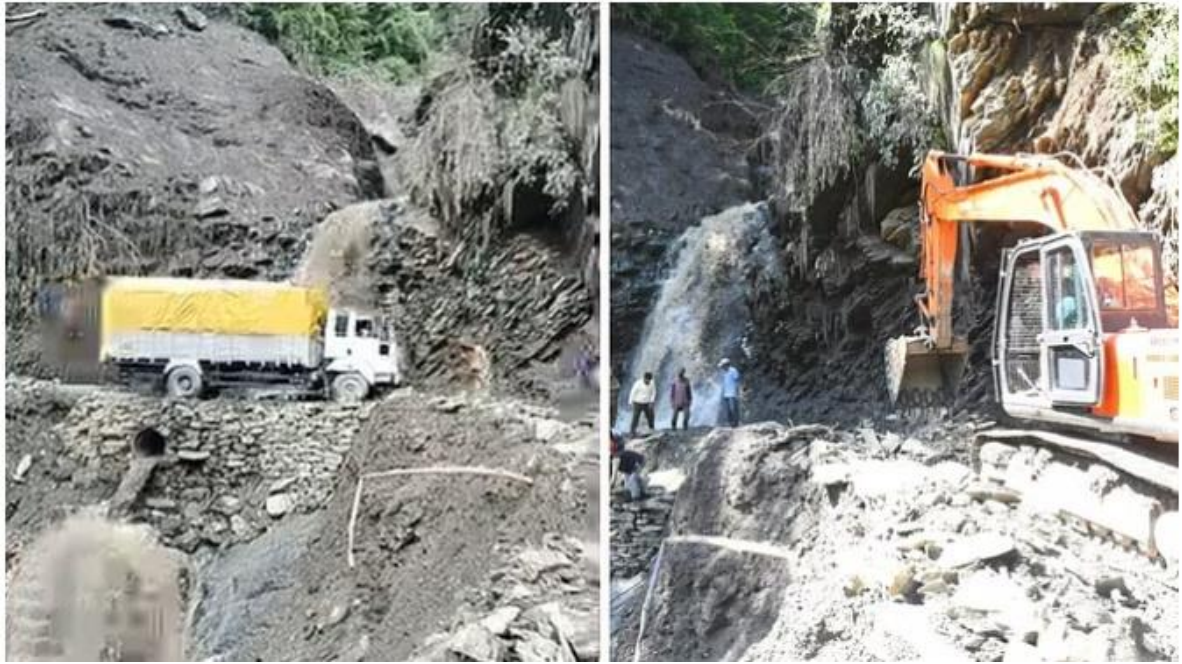
Restoration of road from Taklech to Rampur
