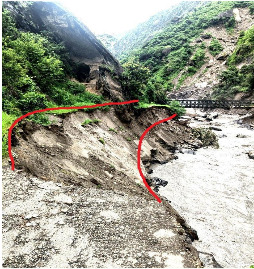
Figure 1 Approach Road to Ganvi Power House Stage-I
