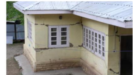
Fig. 2.2.1.3. Impact on opening
