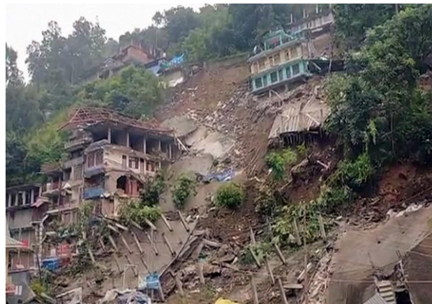
Fig.2.2.2.2 Damage to whole building due to high impact force
