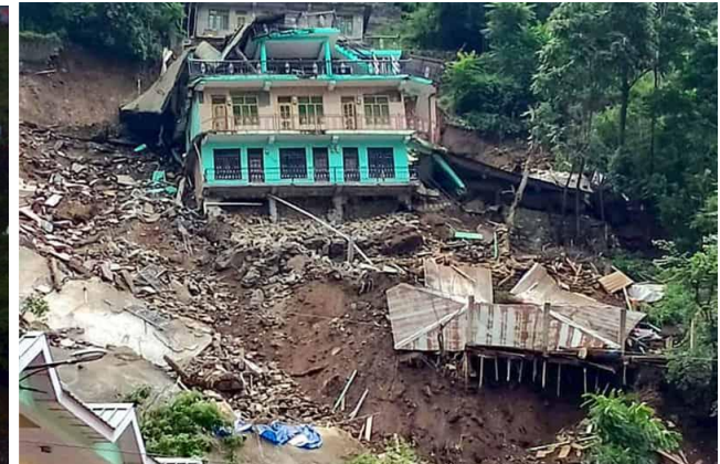
Fig 2.2.2.1. Damage to sub structure due to soil erosion
