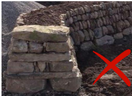
Fig 4.5 Toe Wall Backfill
