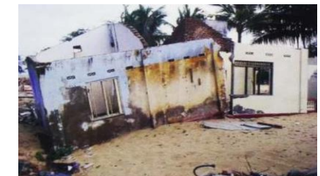
Fig. 2.2.1.5. Impact due to soil liquefaction
