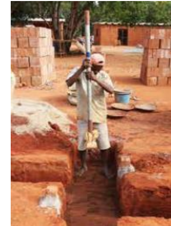
Fig 6.3.1.3. Ram the foundations.
