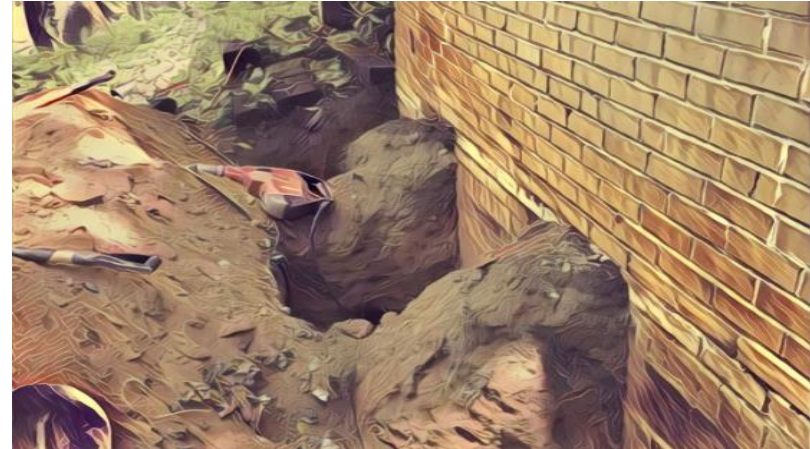
Fig. 6.2.18 Stone in foundation trenches
