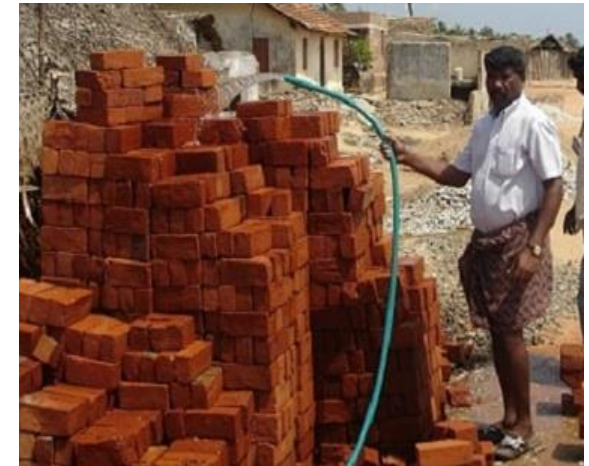
Fig. 6.2.7 Spraying water on Brick stacks
