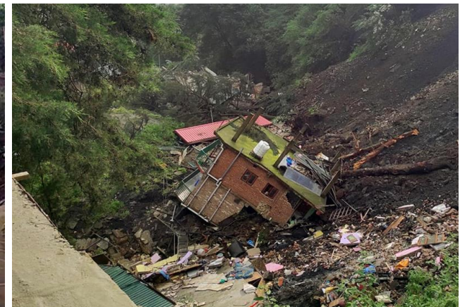
Fig.2.2.2.3. Collapse due to sliding force
