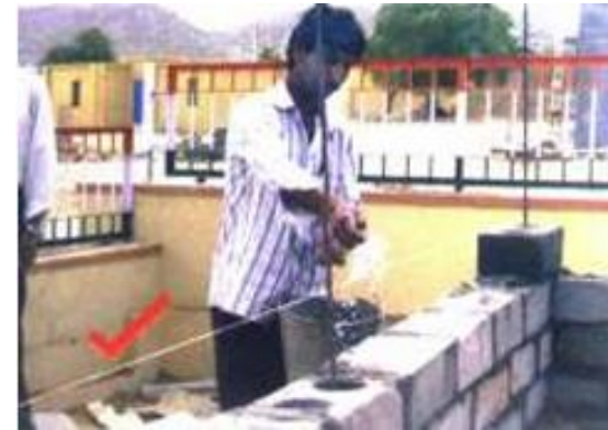
Fig 7.4.6. Water curing cement mortar
