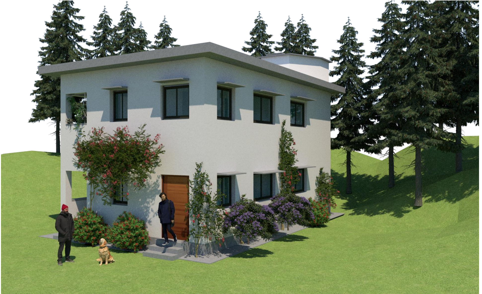
Figure 6.2.1.32. View of the house
