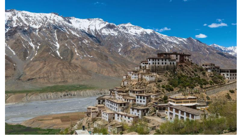
Fig 2.3.1.2. Traditional houses prone to damages from earthquakes, winds, snow, rains, and ground movements
