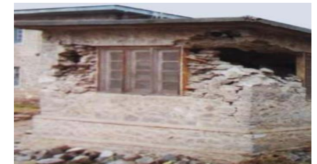
Fig. 2.2.1.4. Impact on corners of the house
