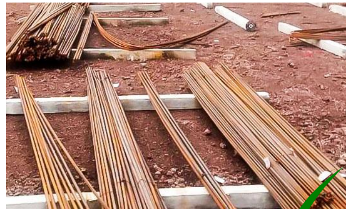
Fig. 7.5.5. Stacking of reinforcement
