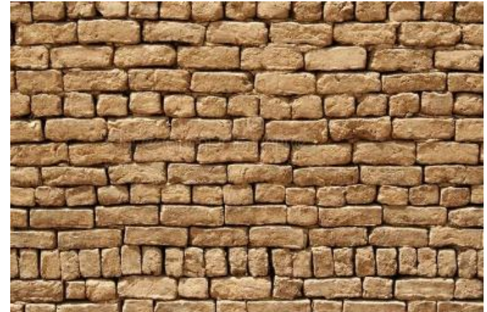
Surface of Mud-brick masonry in cement sand mortar/ RBC roof
