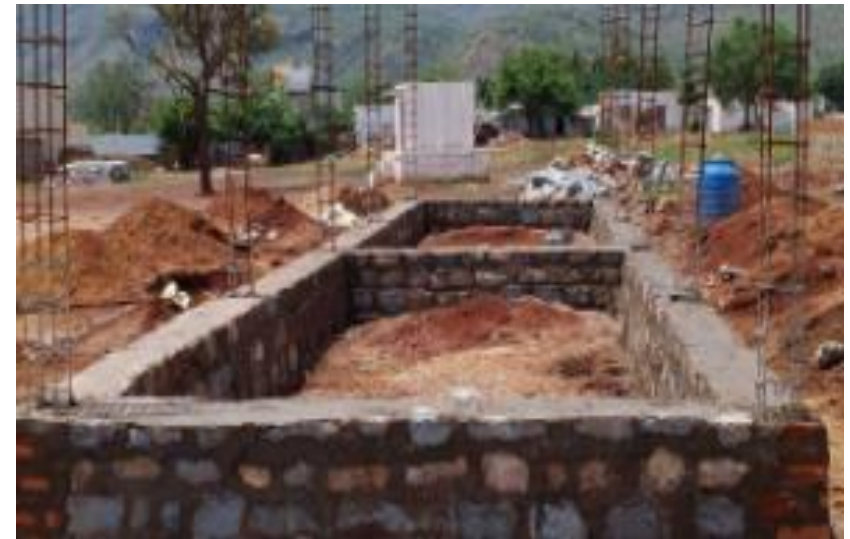
Fig 6.3.1.8. stone masonry in Confined Masonry System
