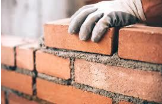
Fig 7.4.1. Mortar thickness wrt brick course
