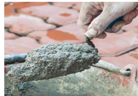
Concrete should neither be harsh nor flowing
