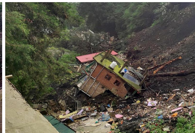
Fig.2.2.2.3. Collapse due to sliding force
