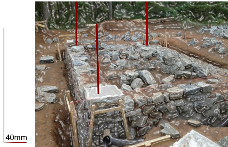
Fig.6.2.22. Boulders fixed in the soil.
