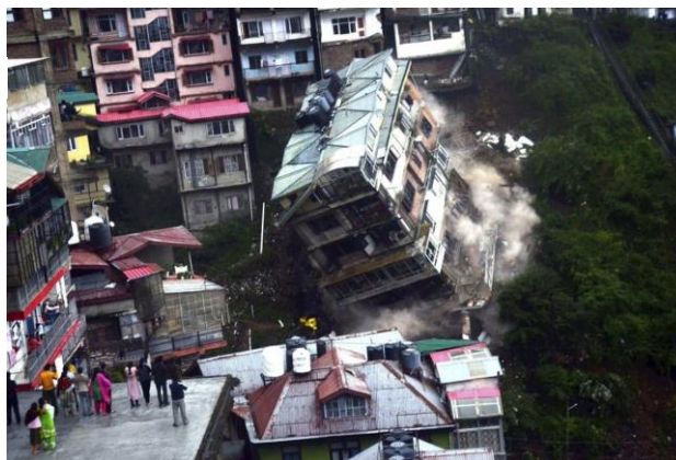
Fig 2.2.2.1. Damage to sub structure due to soil erosion
