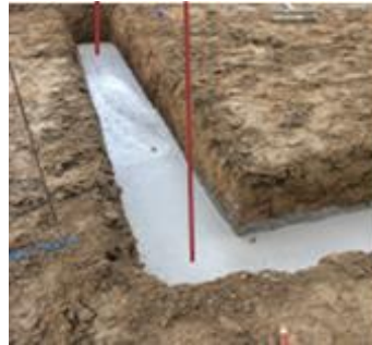
Fig 6.2. 18. Base concrete 120mm
