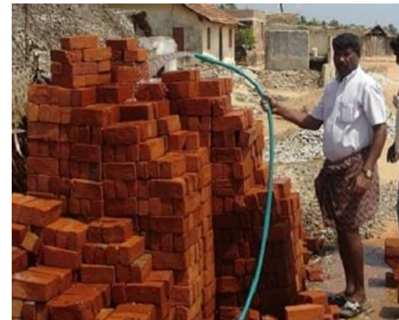
Fig. 6.2.7 Spraying water on Brick stacks
