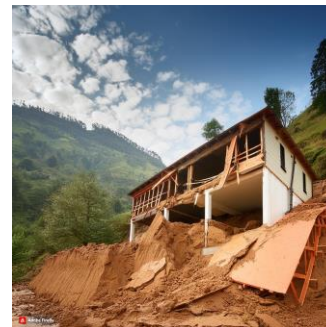
Fig.2.2.3.5. Settlement of foundation
