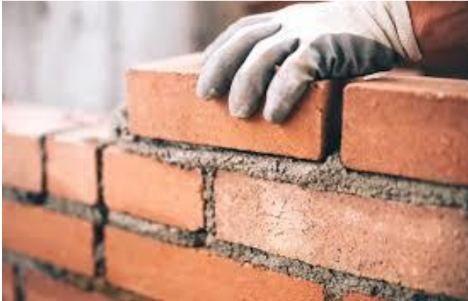
Fig 7.4.1. Mortar thickness wrt brick course
