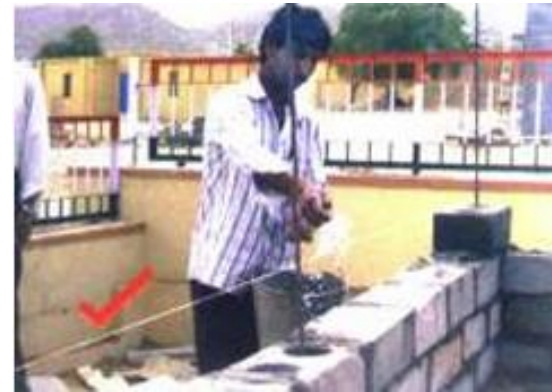
Fig 7.4.6. Water curing cement mortar
