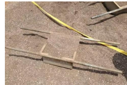
Fig 7.2.4. Measure sand by standard measuring box
