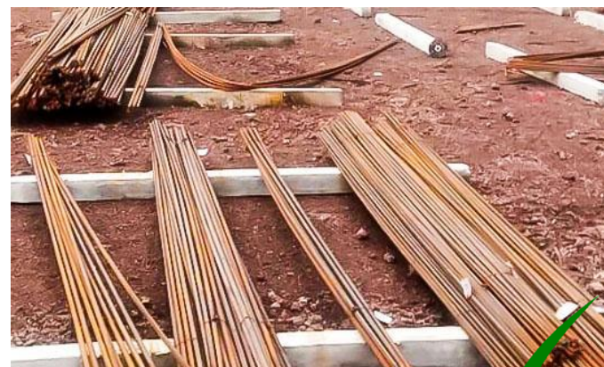
Fig. 7.5.5. Stacking of reinforcement
