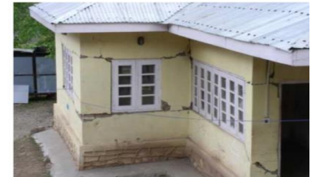
Fig. 2.2.1.3. Impact on opening
