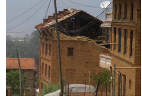
Fig. 2.2.1.2. Impact on gable wall
