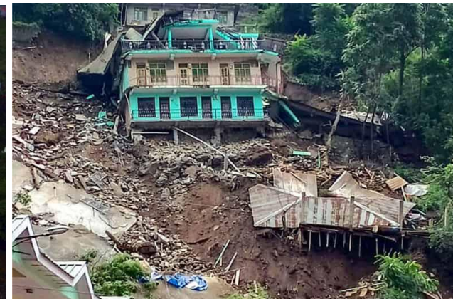
Fig 2.2.2.1. Damage to sub structure due to soil erosion
