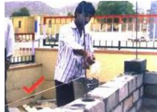
Fig 7.4.6. Water curing cement mortar
