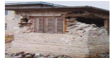
Fig. 2.2.1.4. Impact on corners of the house
