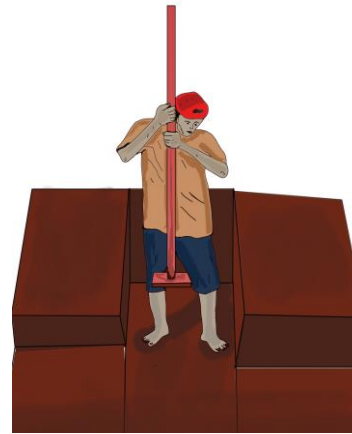
Fig.6.2. 20. Ram the foundations.
