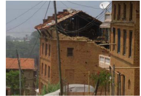
Fig. 2.2.1.2. Impact on gable wall
