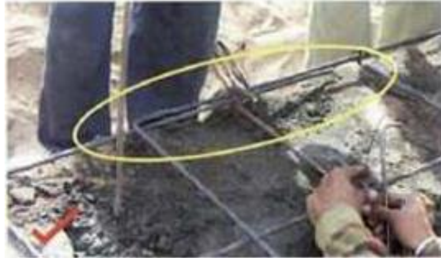
Fig. 7.5.4. Right connection of rod
