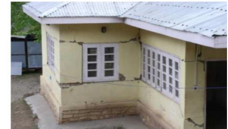
Fig. 2.2.1.3. Impact on opening
