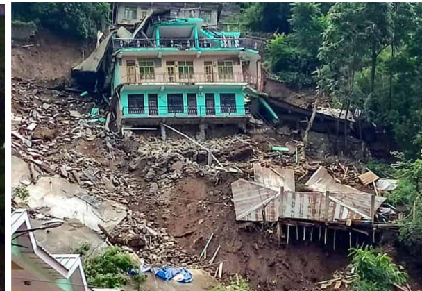
Fig 2.2.2.1. Damage to sub structure due to soil erosion
