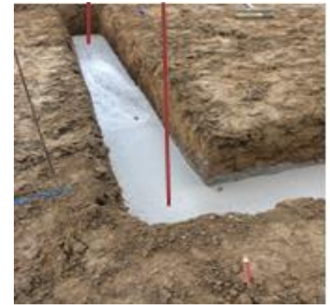
Fig.6.2.21. Base concrete 120 mm.
