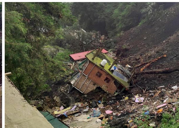
Fig.2.2.2.3. Collapse due to sliding force
