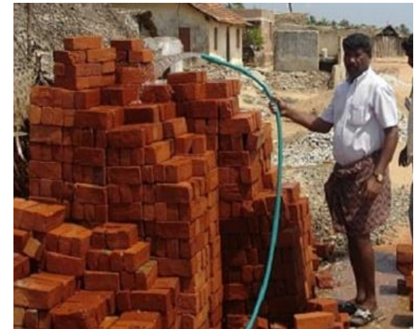
Fig. 6.2.7 Spraying water on Brick stacks
