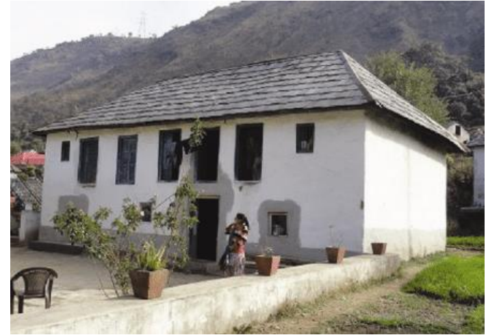
Fig 2.3.3.2. Increasing use of less wooden reinforcement and inadequate mortar in traditional houses makes them vulnerable to earthquakes, winds, rains
