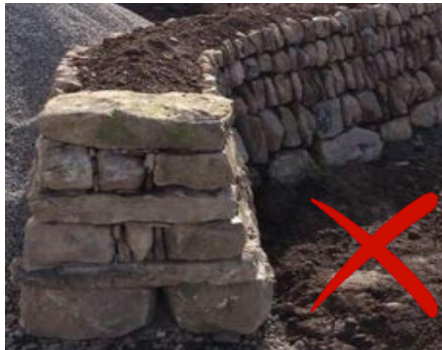
Fig 4.5 Toe Wall Backfill
