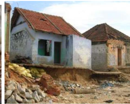
Fig.2.30. Excessive rainfall and splashing may cause the material to lose their properties
