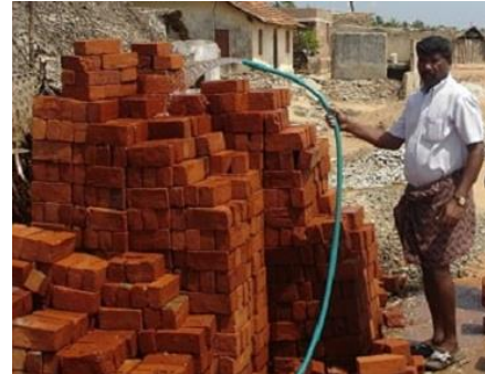
Wetting of bricks prior to construction of walls is imperative
