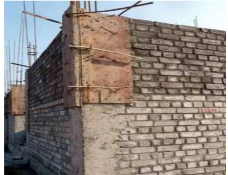
Fig. 3.2.2. Shuttering in confined masonry using Mud bricks
