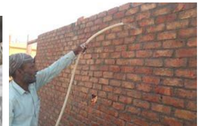
Water curing to be done
