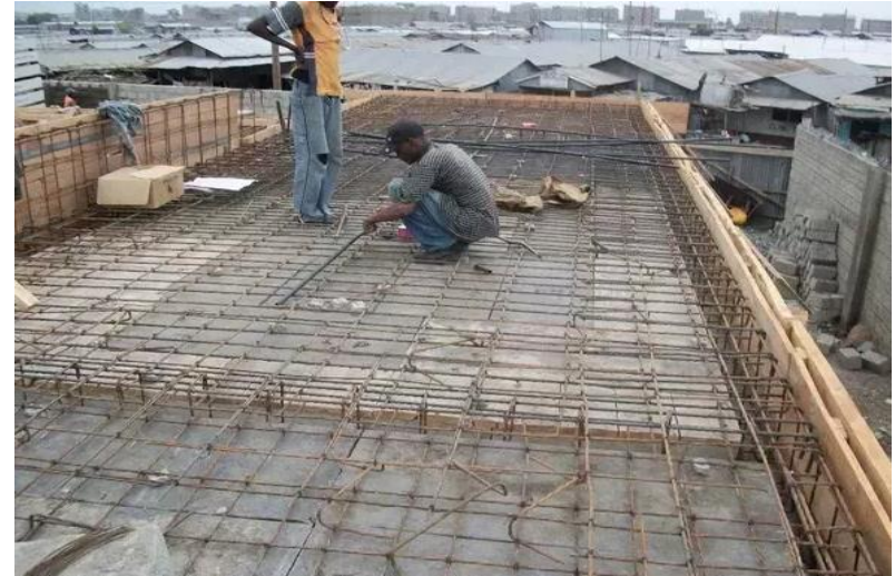
Fig.6.3. Reinforcement being laid on shuttering
