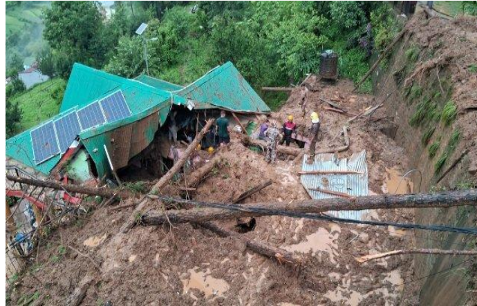
Fig. 2.17. Damage to whole building due to high impact force
