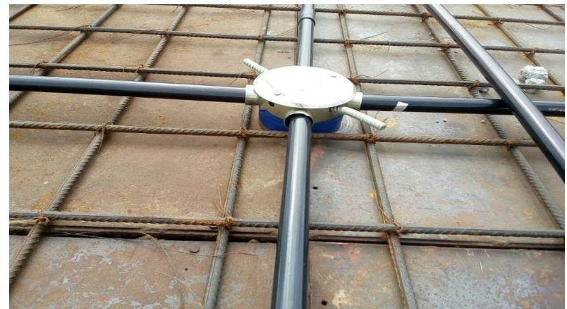
Fig.6.4. Provision of conduits and fanboxes while shuttering is placed
