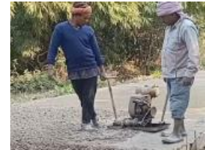
Fig.6.7. Vibrator for compacting
