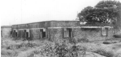
b) A building with horizontal lintel band in Killari village survives
