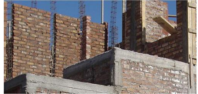
Fig. 3.2.1. Confinement in masonry using mud bricks
