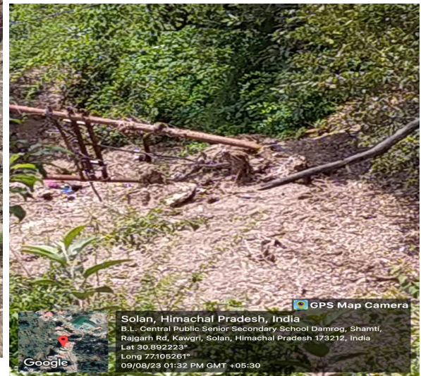
Figure 5 Fully washed out and found nearby place
