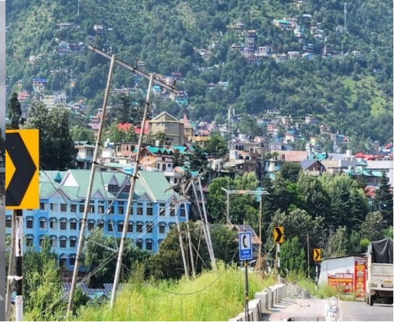
Figure 10. Poles Deformity of Structures Due to
