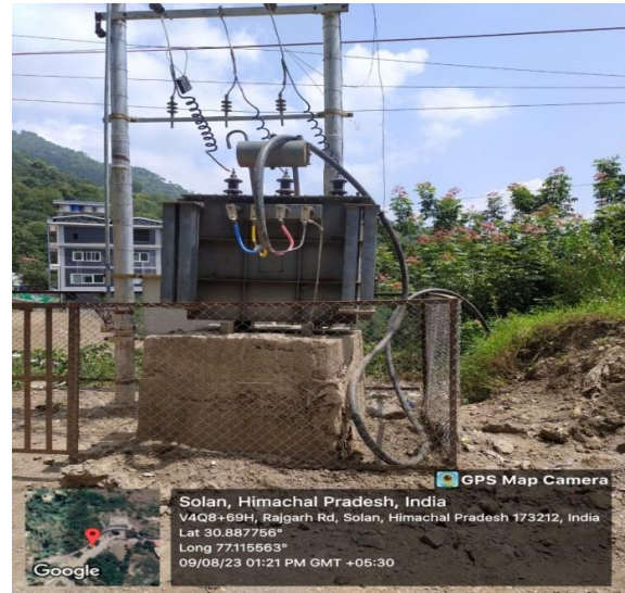
Figure3 Location after restoration
