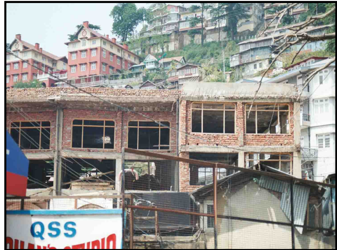
Common Structures .in Himachal Pradesh
