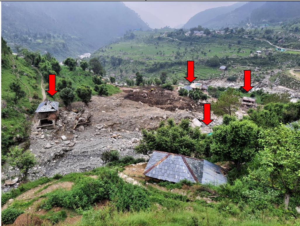
Photo-5: The downhill view of debris flow hit Boh village with remains of damaged houses (shown with red arrows)
