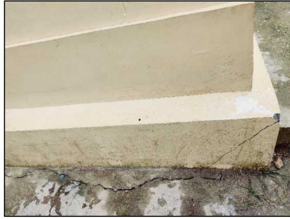
Fig. 36. Cracks developed in the newly constructed school building (just before monsoon).
