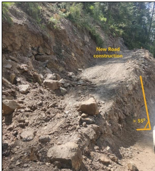
Fig. 33. New Road construction with large slope angle.
