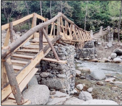
Fig. 35. Temporarily constructed bridge.
