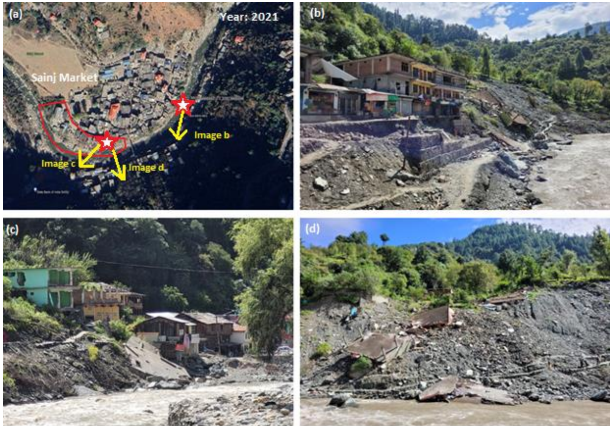
Fig. 17. Near Sainj Market, a landslide caused subsidence of ground by around 1.5 meters over a 50 meter area, resulting in displacement of the retaining wall intended to provide slope stability. The root zone stability of the orchards has been impacted.
