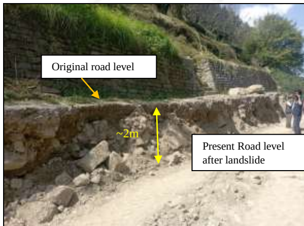
Fig.29; Ground cracks along the lower most road level at Bandal.
