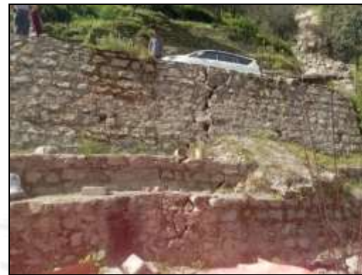
Fig.30 ; Damaged retaining wall towards valley side of lowermost road level.
