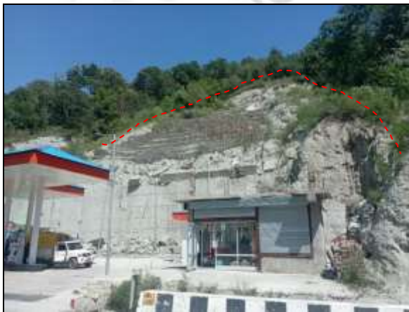
Fig.7; Debris slide on upslope of Indian oil petrol pump.
