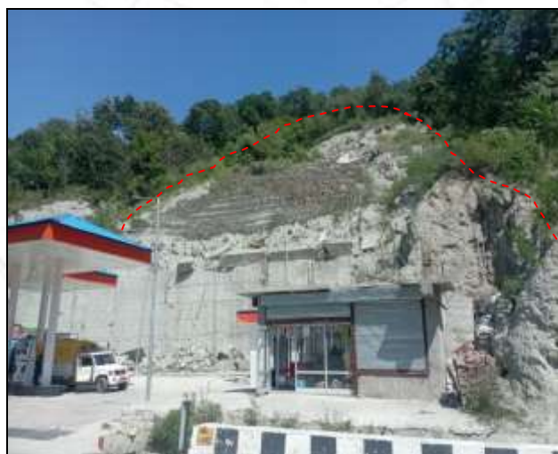
Fig.1. Debris slide on upslope of Indian oil petrol pump
