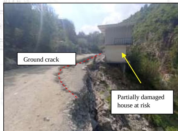
Fig.41; Ground cracks and House at risk located towards valley side of the road along Thana Sainj to Taxi stand road stretch.
