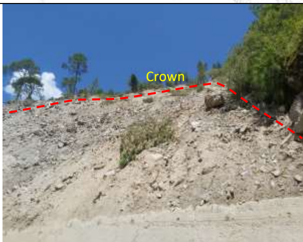
Fig.79. Unstable crown portion of slide
