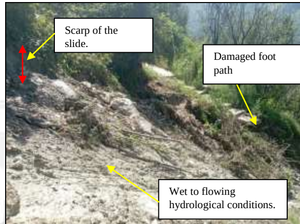
Fig.11; Main body of the landslide.
