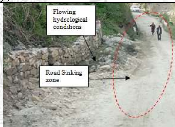
Fig.3. Road subsidence
