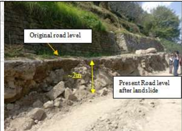
Fig.3. Road subsidence
