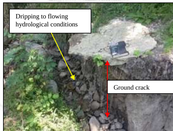
Fig.9; Seepage zone in flowing water conditions along ground cracks in the distressed slope.
