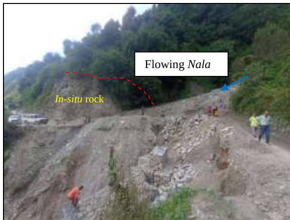
Fig.17; Right flank of Garsa village affected slope.
