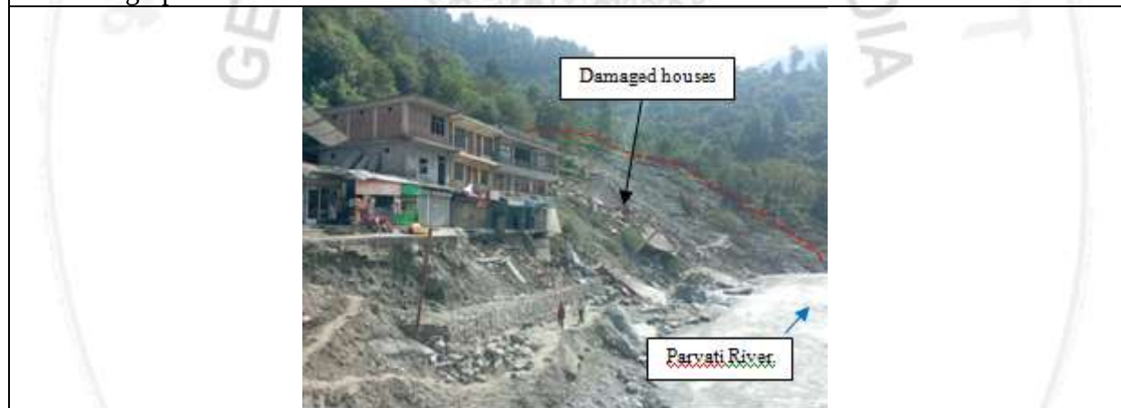
Fig.1. Main landslide affected are
