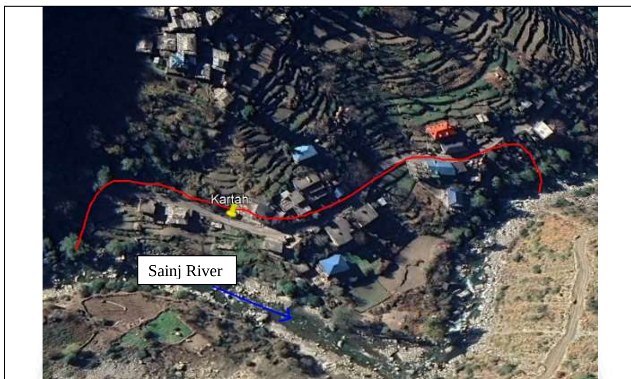
Fig.1. ; Kartah subsidence (Source: Google image)
