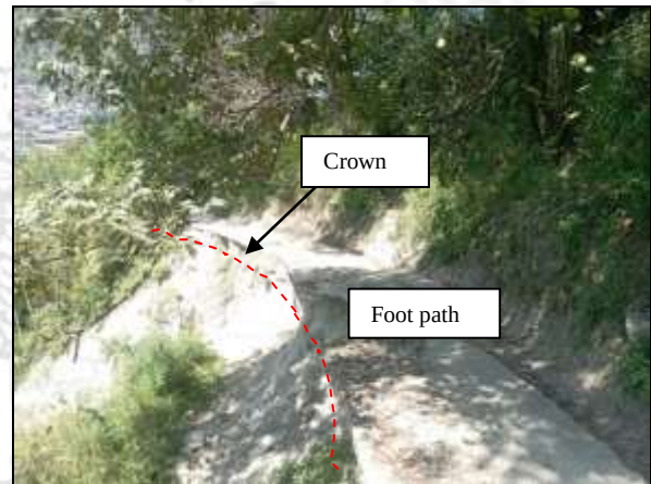
Fig.8; Crown of the landslide.
