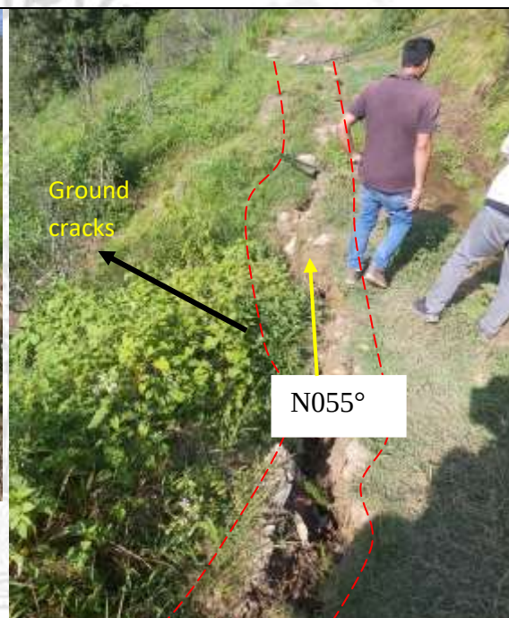
Fig.2. Open ground cracks in Chehava slide
